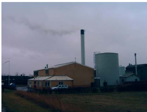
Fig. 4: CHP plant – notice the accumulator of 655 m3
